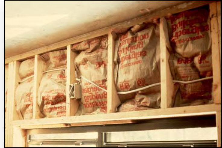
Missing (left) and crushed (right) insulation.
