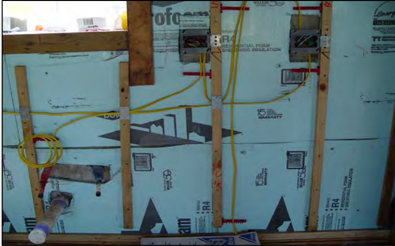
Missing (left) and crushed (right) insulation.
