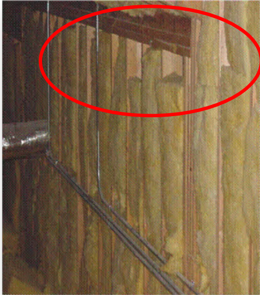
Missing and crushed insulation (left) and infrared photo indicating insulation anomalies (right)
